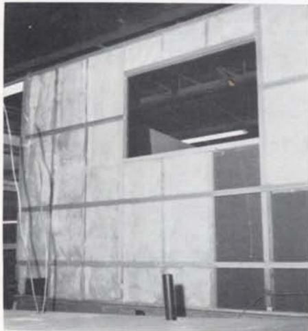
View of end wall showing thick fiberglass insulation and furring strips.
